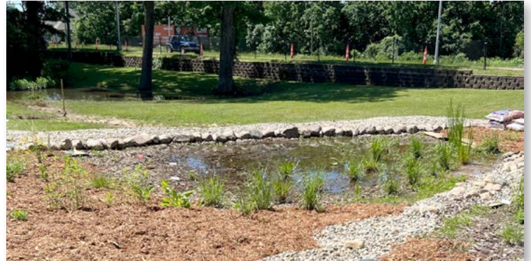
A rain garden holds water in a shallow "bowl" allowing it to be slowly absorbed. The deep-rooted native plants filter many of the toxins contained in the water before it reaches the watershed.
