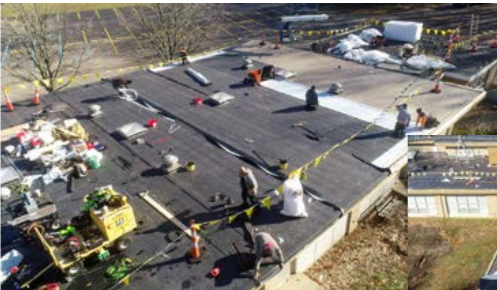
(Above and right) The roofing crew at work installing the insulation material (white) and the EPDM roofing membrane (black layer), designed to last 30+ years.
