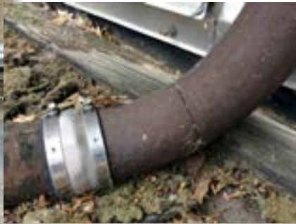
Pipes installed on the old roof to aid in proper drainage were rusted, cracked and failing.
