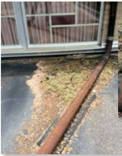
Pipes installed on the old roof to aid in proper drainage were rusted, cracked and failing.
